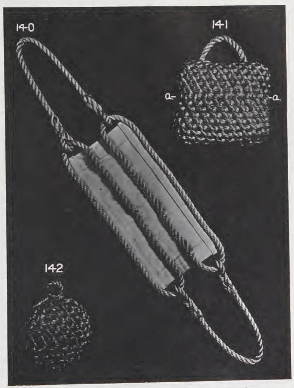
PLATE 253-A SLING, AND TWO TYPES OF FENDERS
