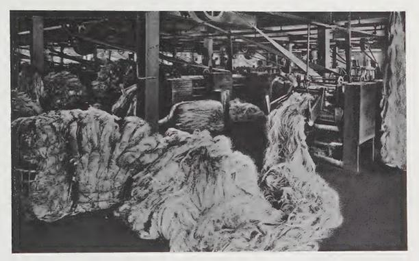
In the preparation department of the cordage mills the bales of fiber are opened and the "hemp" is put through a series of operations, to straighten and parallel the fibers, until a small even ribbon of "sliver" is finally produced.
